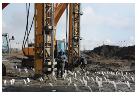
Figura 14 – Câmp de drenuri verticale ( http://www.egezemin.com/fitil-dren )
