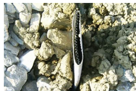
Figura 14 – Câmp de drenuri verticale ( http://www.egezemin.com/fitil-dren )
