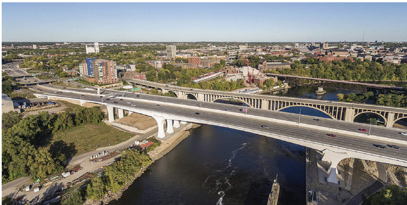
Figura 11 – Podul I-35W, St. Anthony Falls Bridge
