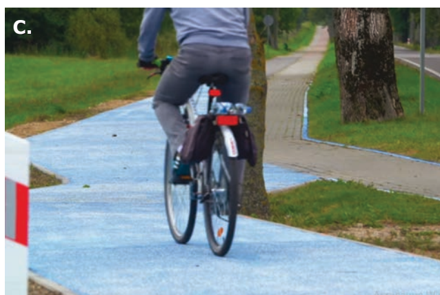
Figure 3. Perspective types of coating for bicycle paths: a - permeable concrete covering; b - permeable asphalt covering; c - coating with a phosphor in the afternoon; d - coating with phosphor at night
