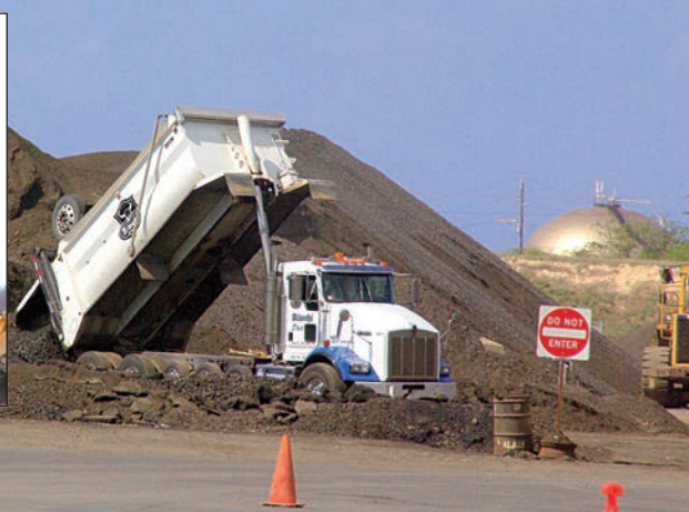
Foto 1: Reclaimed Asphalt Pavement – RAP (Asfalt reciclat)
