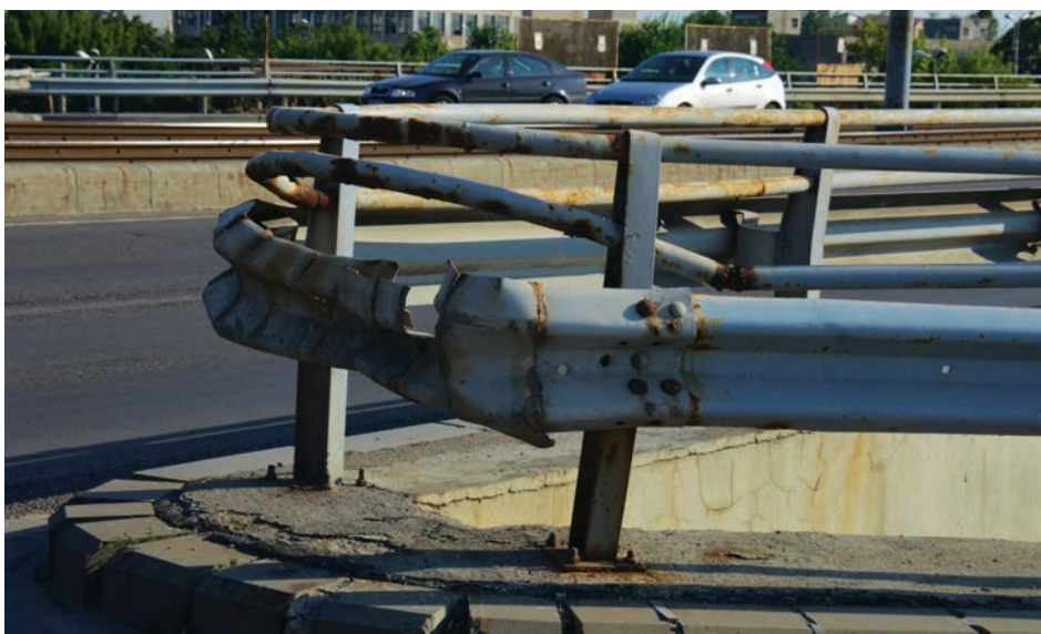
Parapetele metalic – rampa Giulești, “Podul Grant”
