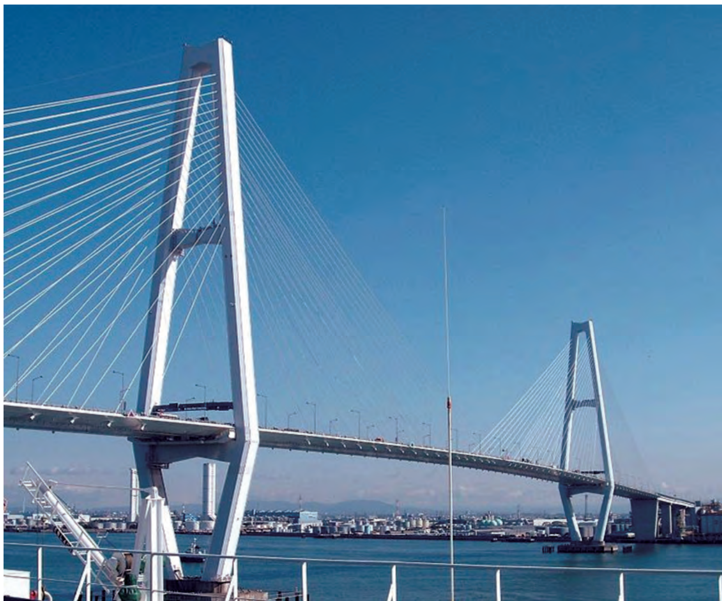
Fig.13 - Meiko-Chuo, cable stayed bridge
