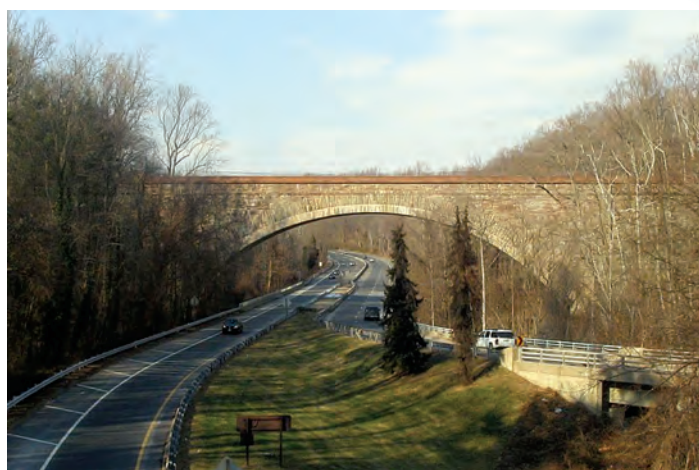
Fig. 1 Union Arch Bridge
