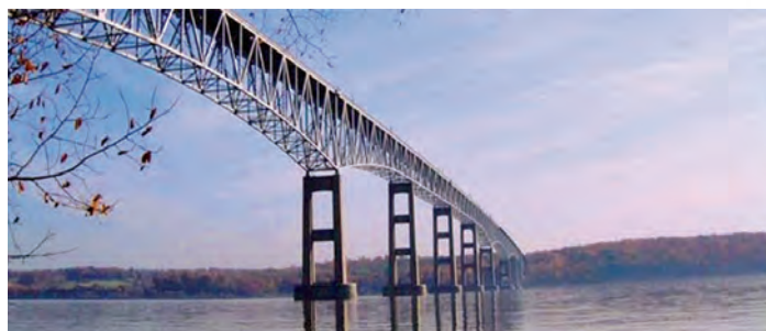
Fig. 2.1 - „Kingston-Rhinecliff Bridge, a continuous under deck truss bridge” (tablier continuu cu zăbrele având calea sus)
