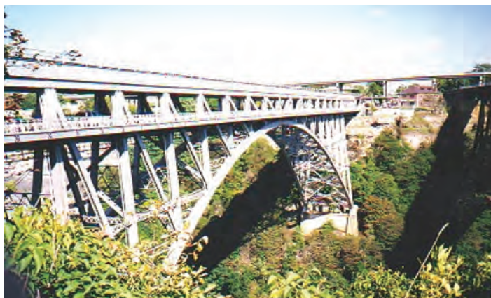
Figura 12 - Lower Steel Arch Bridge (Whirlpool Rapids Bridge)
