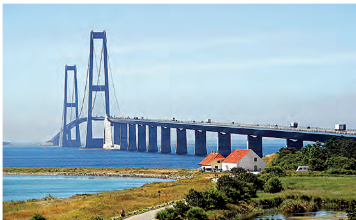
Fig. 6 Podul Great Belt East, Danemarca (deschiderea de 1.624 m, 1997)
