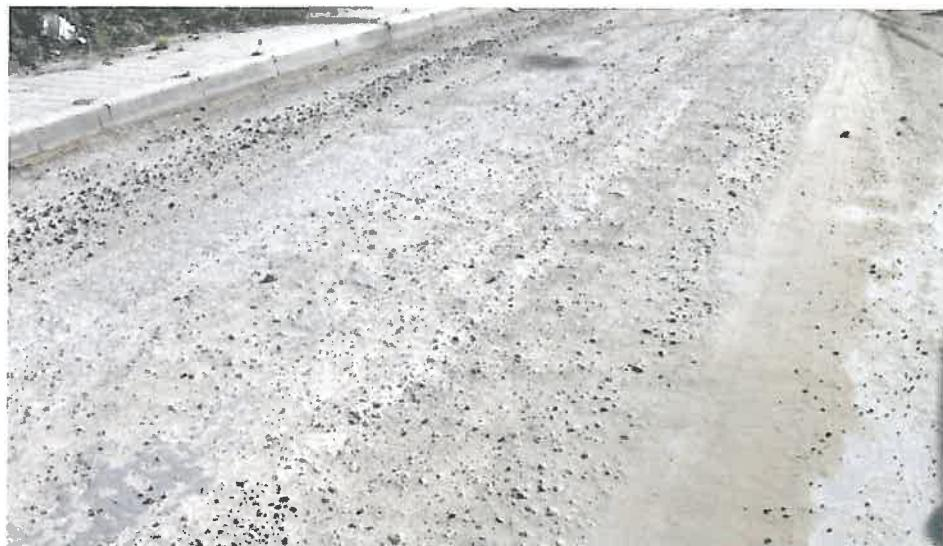
**Figure 9. Visible damage in the recycled material 8 days after opening to traffic**
