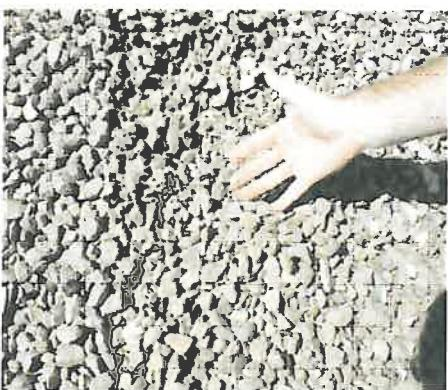
Foto. 4. Tratament incorect, aggregate murdare, neuniforme
